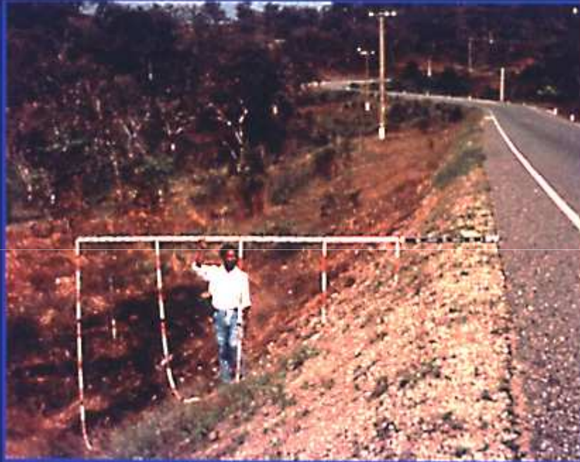
Steep side slope
