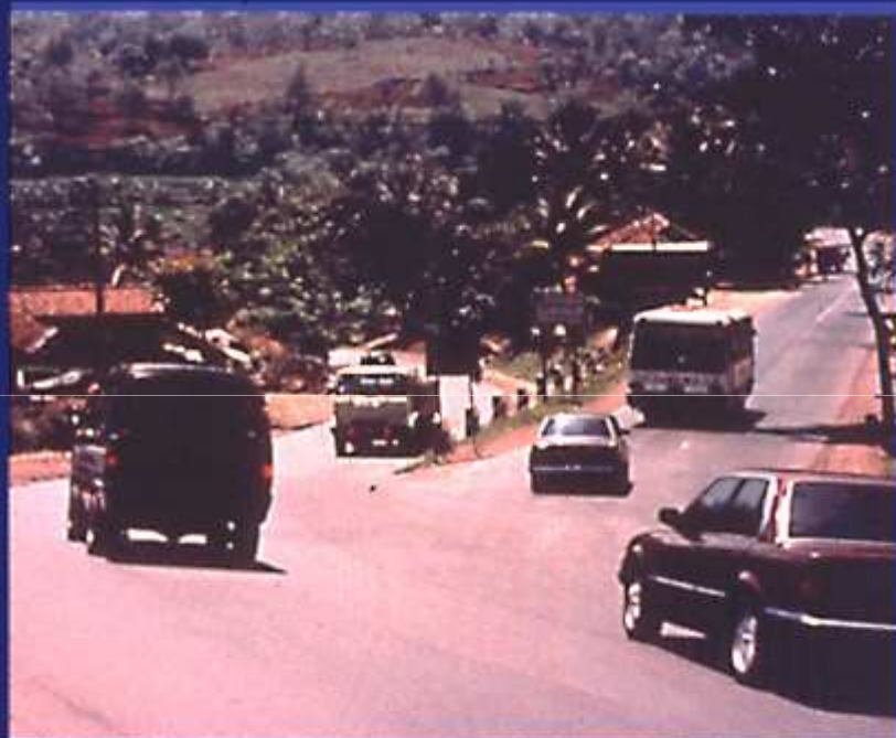
Poorly designed T junction with very poor sight lines
