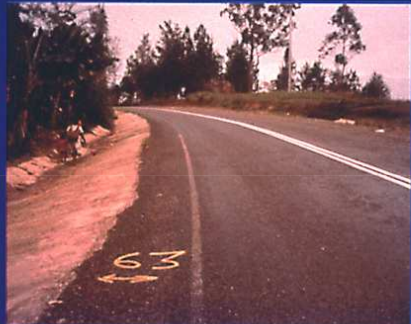
Shallow side slope
